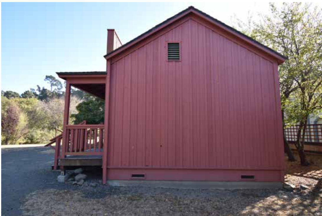
Secondary (North) Elevation of Cambria Chinese Temple South-Facing View; Photo Taken 10/28/2019
