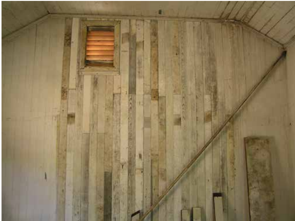
Interior View of Cambria Chinese Temple (South Wall) Following Wall Cladding Repairs and Prior to Paint Restoration Photo Taken Ca 2007
