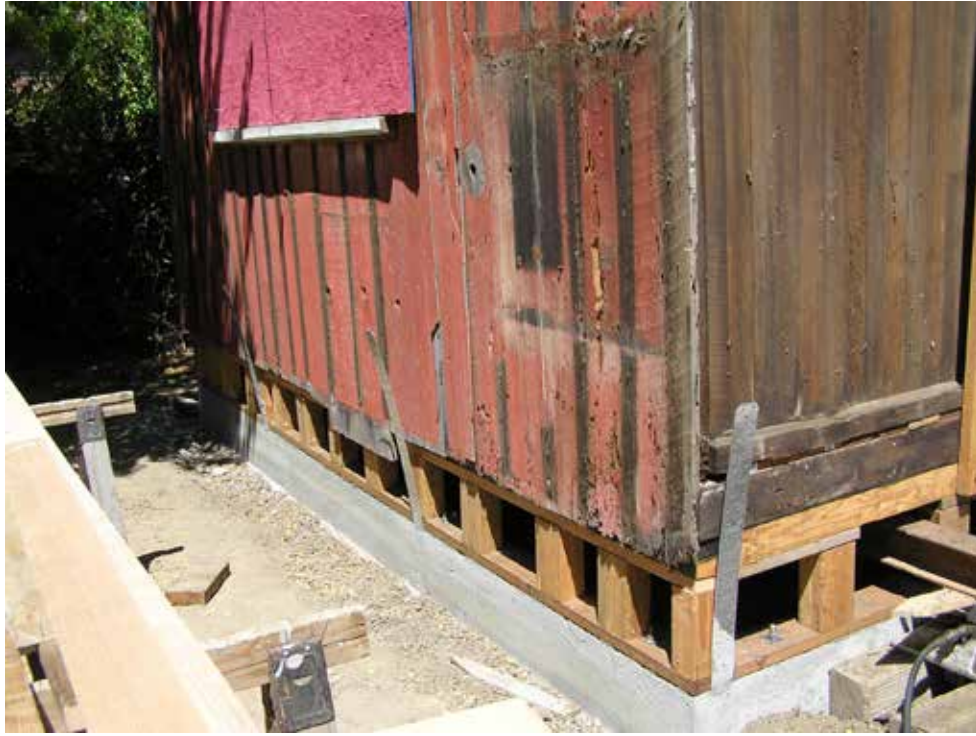
Cambria Chinese Temple Following its placement on New Foundation Photo Taken Ca 2007
