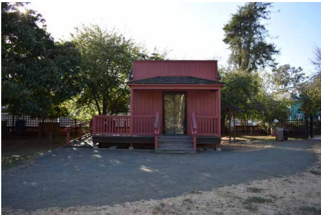
Primary (East) Elevation of Cambria Chinese Temple West-Facing View; Photo Taken 10/18/2019
